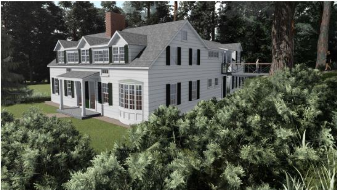
Rendering of the North Shore Land Alliance's new headquarters. Set to open in early 2023.
